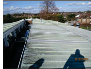
Existing standing seam pitched roof (light green)
